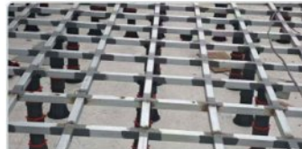
Balcony / WPC Deck
