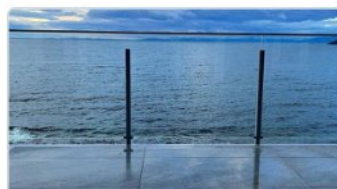
Deck Installation Canada
