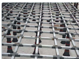
WPC Rooftop Shanghai, China
